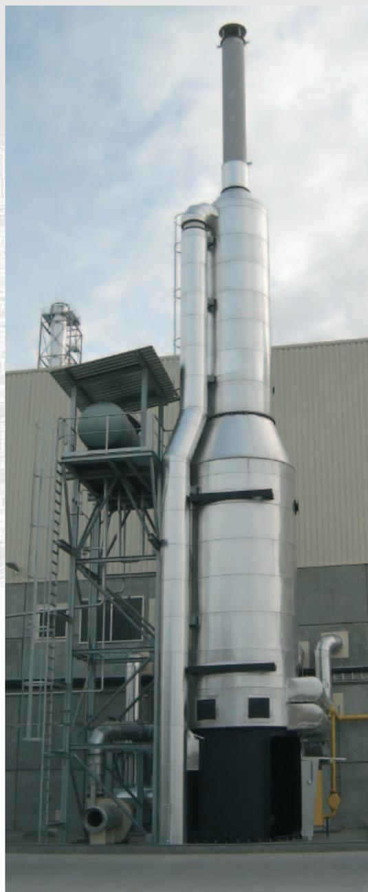
**Heater in vertical layout, capacity: 9.6 MW with built-in combustion air preheater and subsequent stack, total height: 25 m, fired with natural gas; for heating of a particleboard press, Romania**
