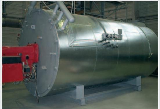
**Thermal oil heater fired with natural gas with a capacity of 1.6 MW, installed in Texas, USA, for the food industry**
