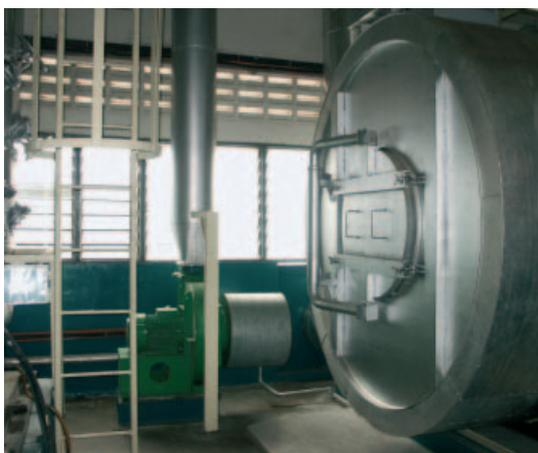
**Horizontal heater with a net capacity of 10 MW with combustion air preheater, fired with light oil entry door at the reversing chamber for the inspection of the combustion area, Malaysia**
