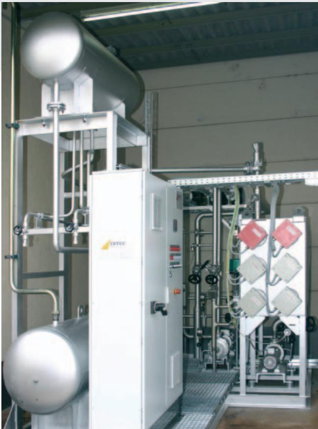
**Electric heater with an output of 150 kW with six heating elements for individual and exact regulation of capacity**
